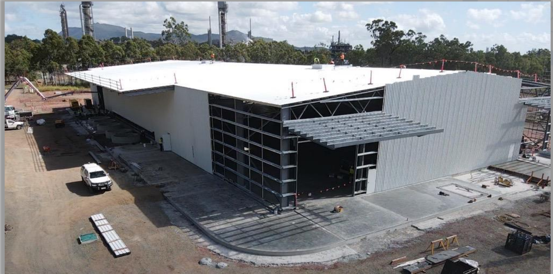
Cladding of the main PPF Building nearing completion
