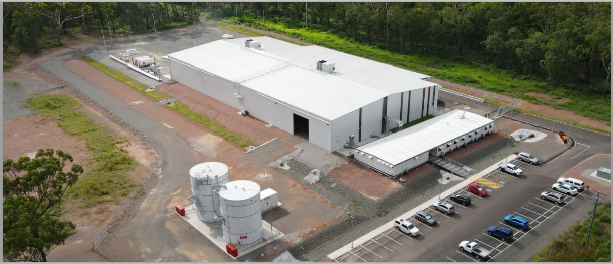
Completed Stage 1 PPF
