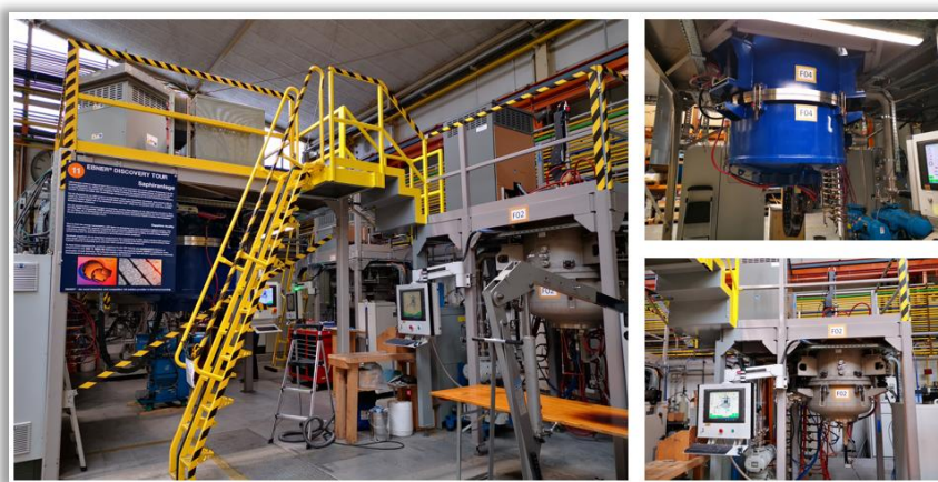
Sapphire crystal growing units at Ebner-Fametec's Austrian facility
