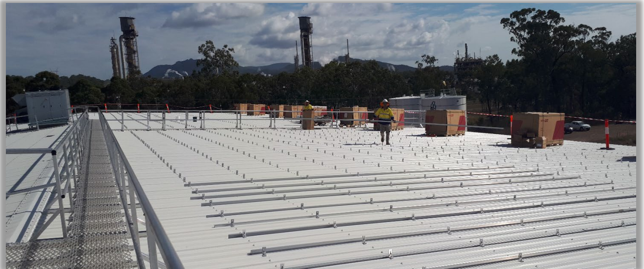
Rooftop Solar Installation – Stage 1 PPF
