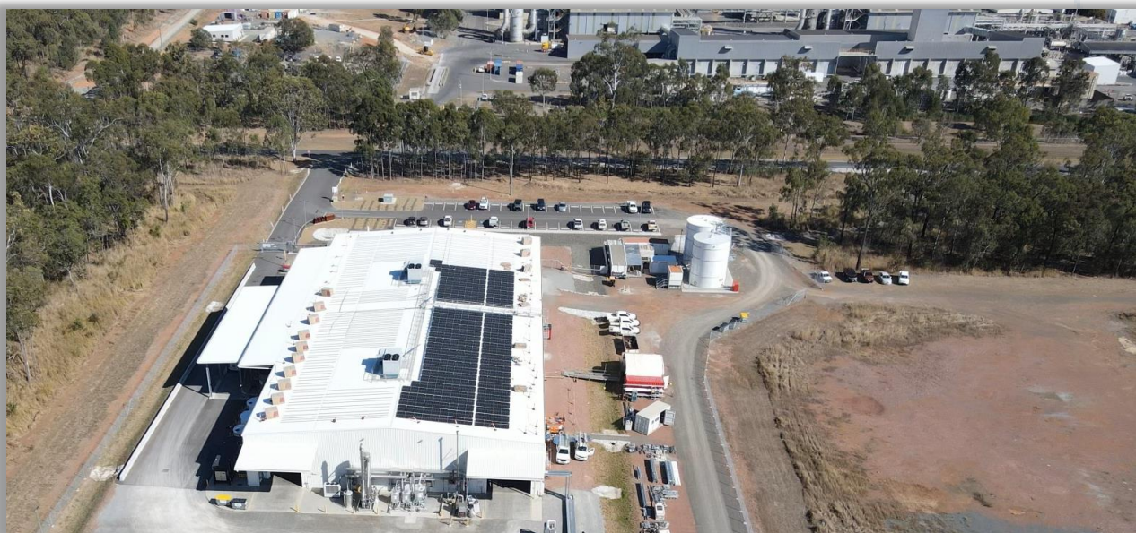
Stage 1 PPF – showing rooftop solar installation
