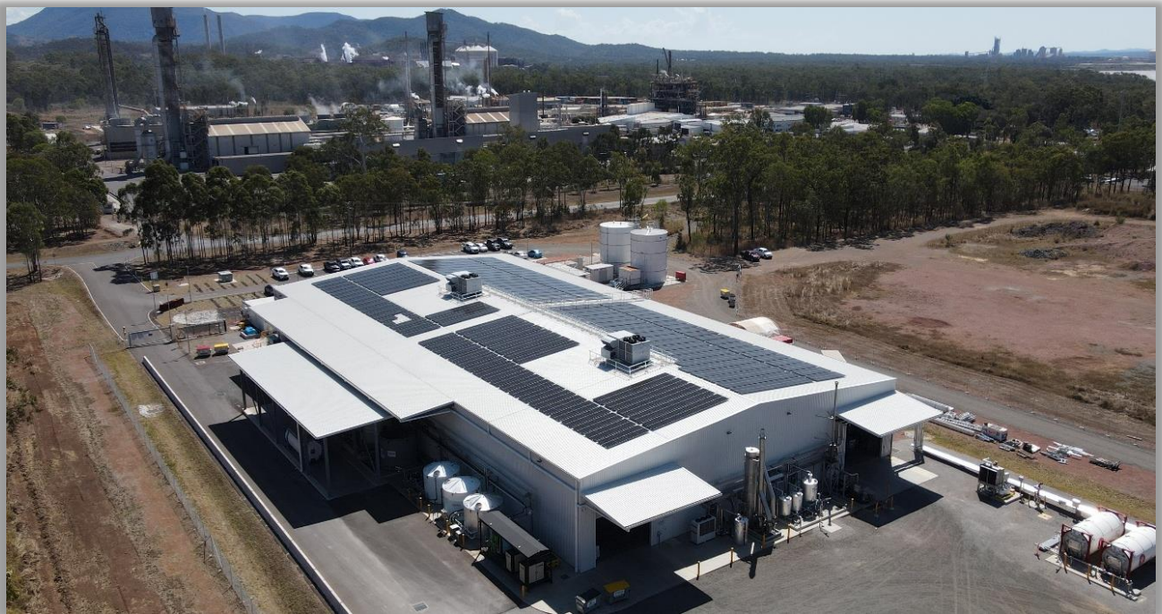
Stage 1 PPF – showing completed rooftop solar installation
