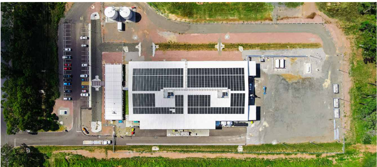
Rooftop Solar Installation – Stage 1 PPF
