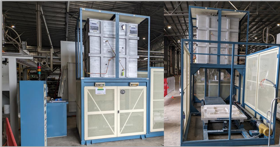
Sinter oven for HPA tablets – under electrical installation
