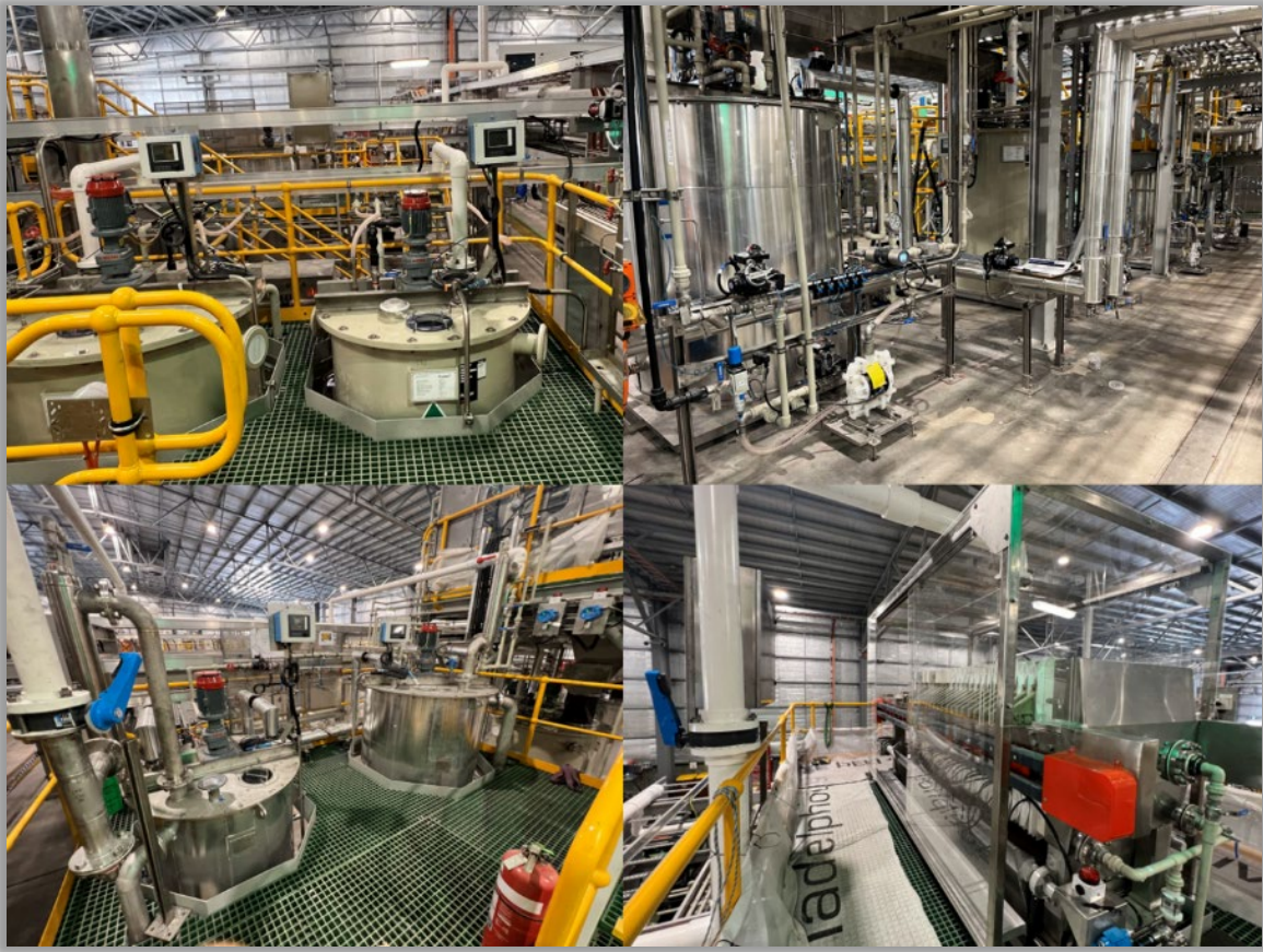
Area 1270 (high-purity boehmite and alumina trihydrate) circuit – under commissioning.
