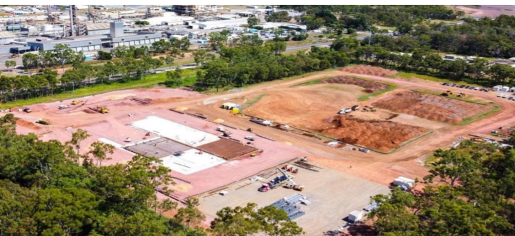
► Stage 1 PPF - preliminary earthworks
