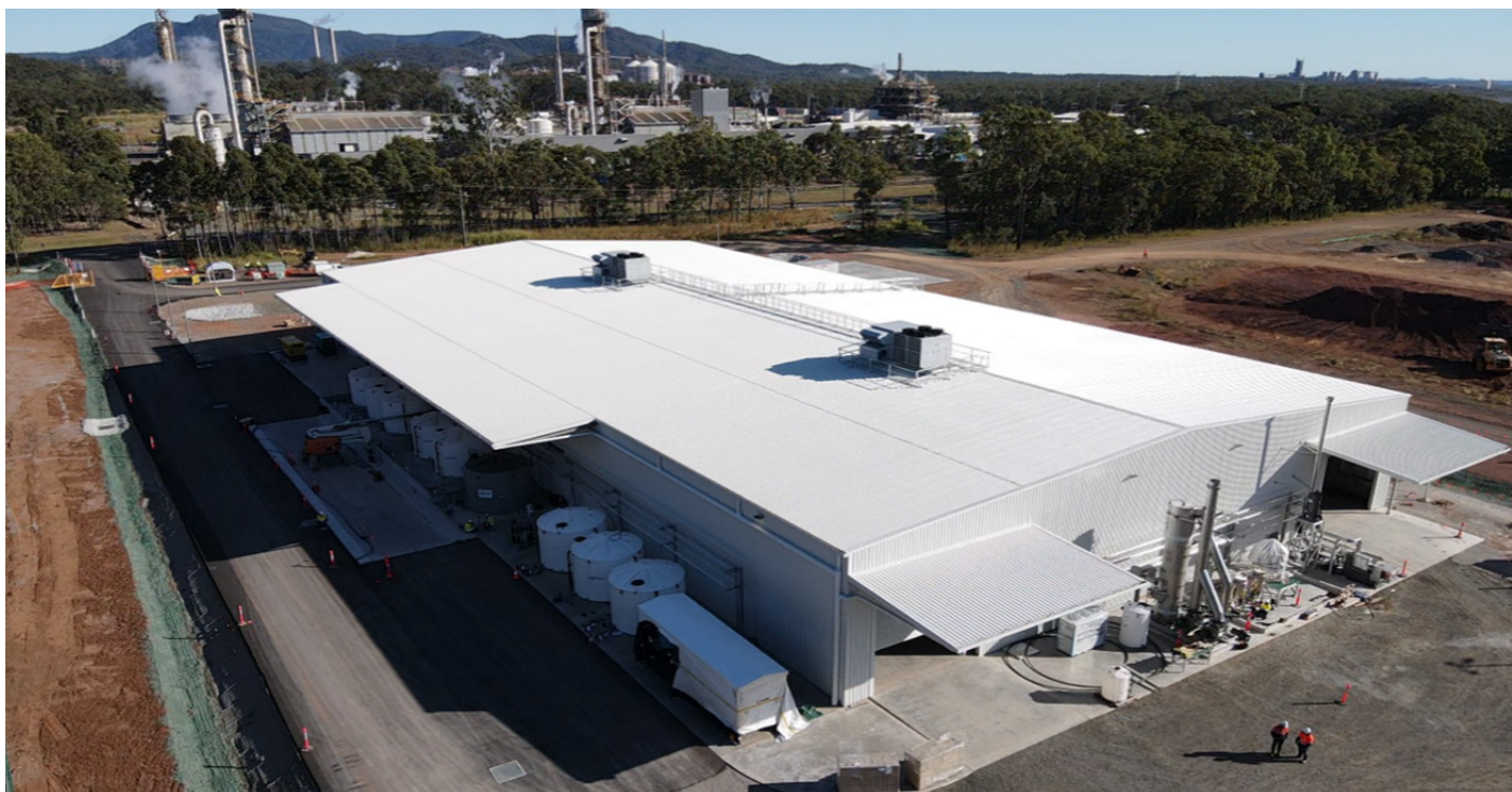
► Stage 1 PPF building at lockup stage
