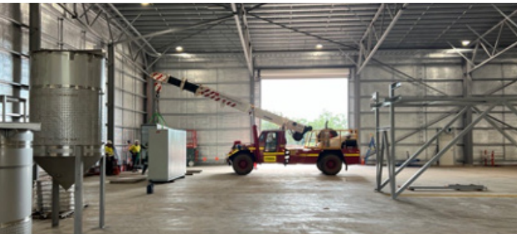
► Interior lighting installed and energised with process equipment deliveries continuing
