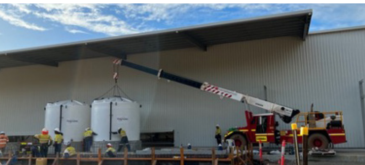
► Installation of PPF reagent tanks
