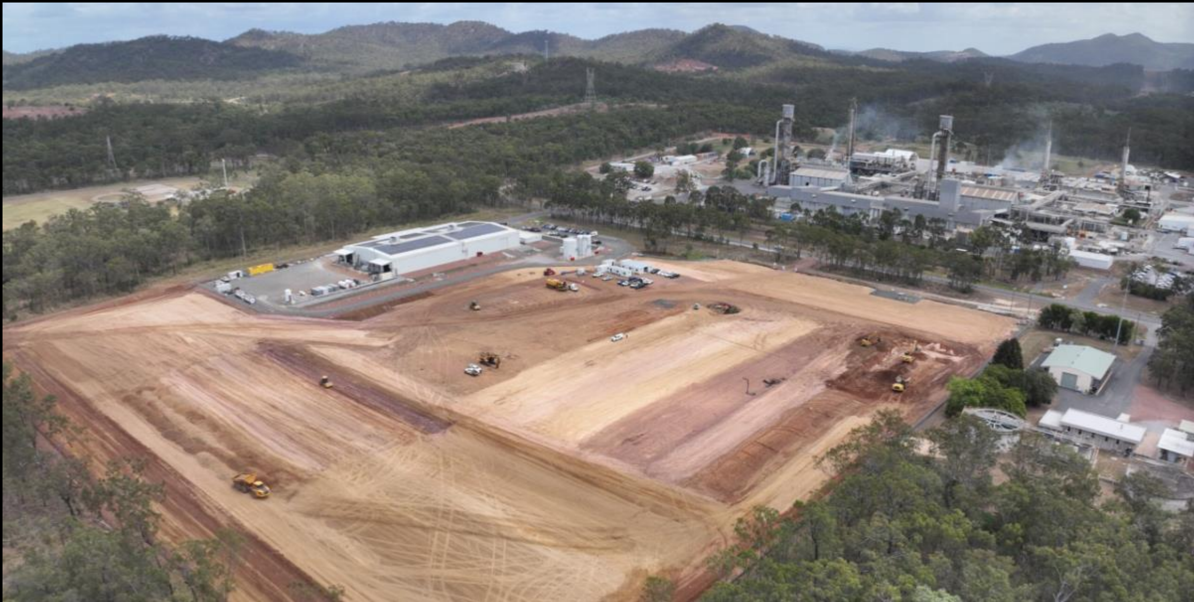
Stage 2 Earthworks – September 2024
