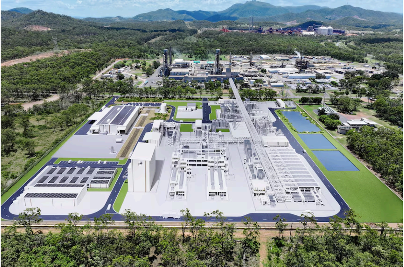
A render of the HPA First Project, due to be complete by next year. (Supplied: Alpha HPA)
