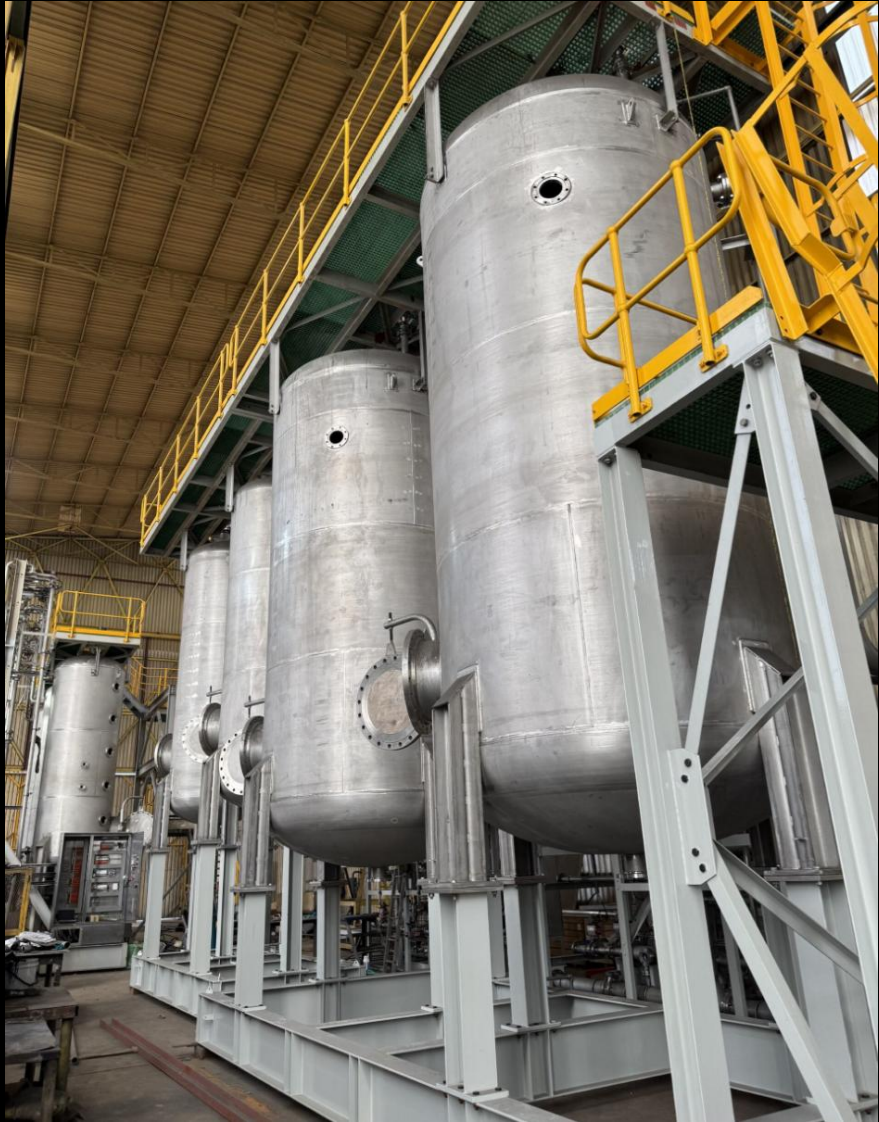
Carbon Columns Assembly Test
