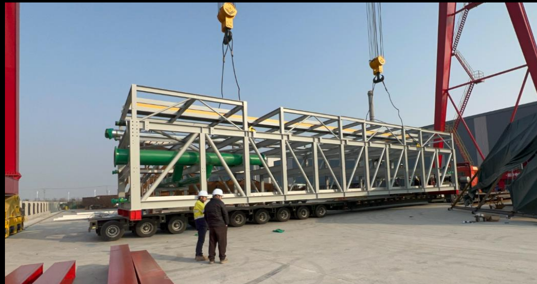
Pipe Rack Assembly
